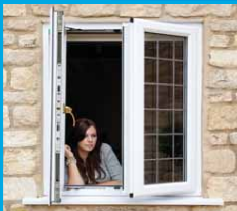
Multiple window openings (French Casement) - Double side hung, opening outwards.
